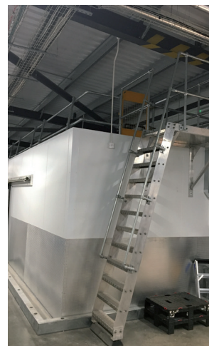
Companionway / Ships ladder with top platform
